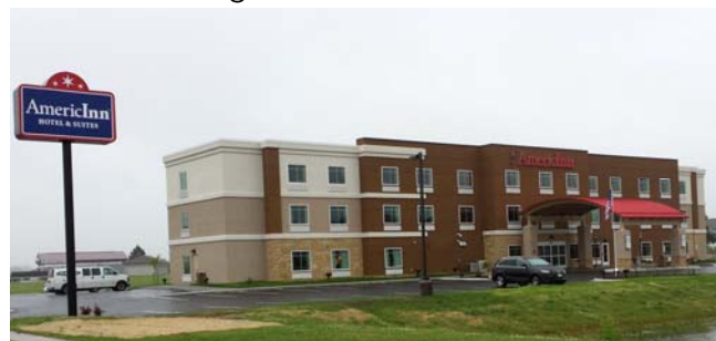
The new 61-bed AmericInn Hotel & Suites, located on Shaler Drive.
