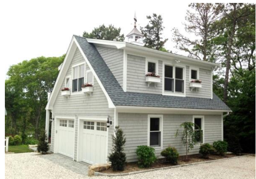
Accessory Dwelling Unit above a garage.
