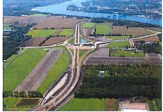
Construction completion anticipated in 2018
